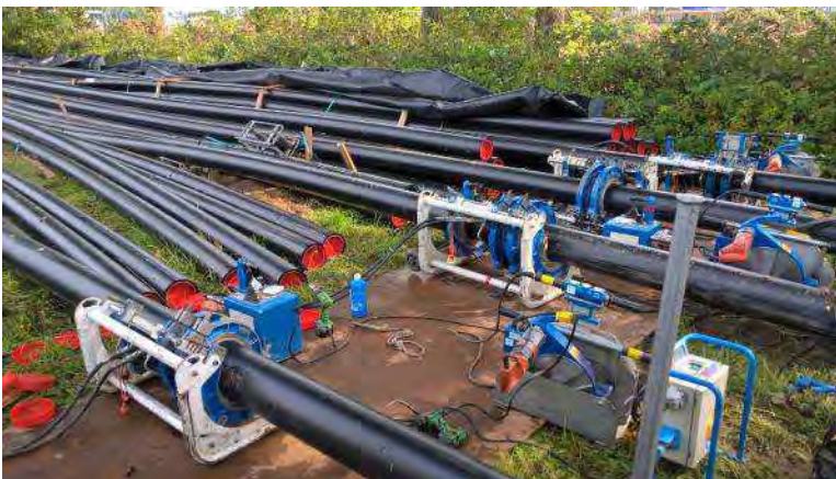
Figure 27 Welding of HDPE ducts
