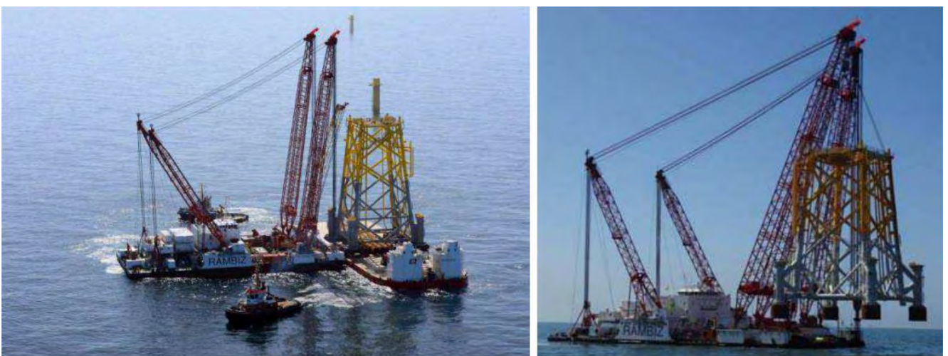
Figure 58 Installation of jacket
