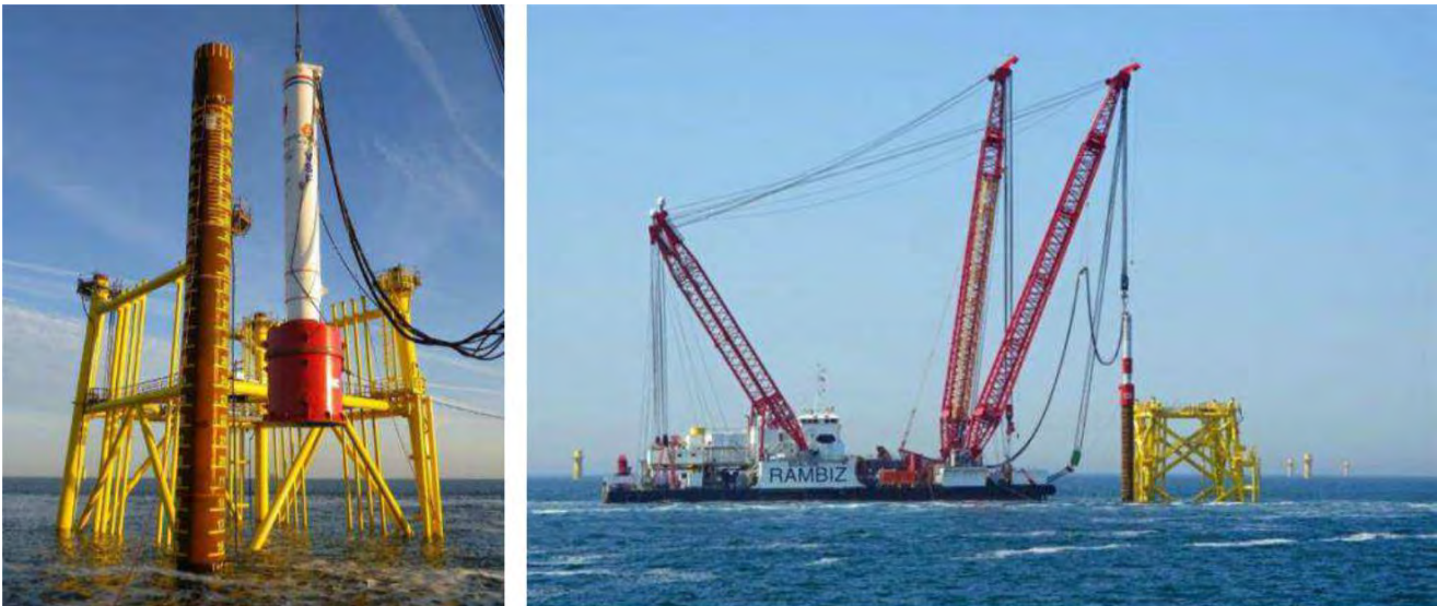
Figure 59 Piling of jacket
