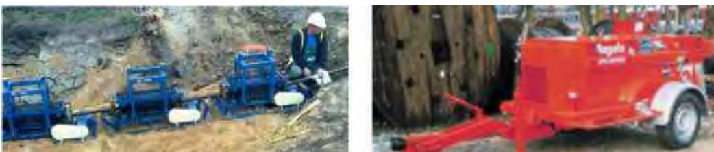
Figure 17 Typical cable tensioners (left) & cable winch (right)
