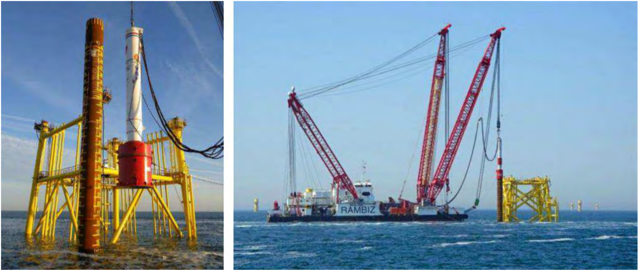
Figure 59 Piling of jacket
