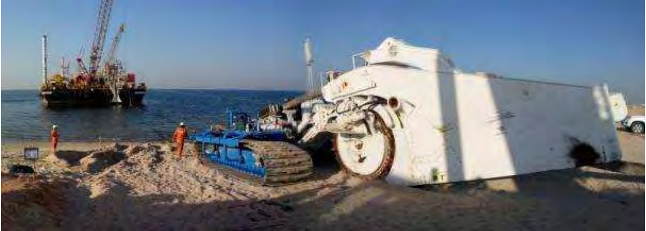
Figure 41 TM04 Wheel cutter cable trencher
