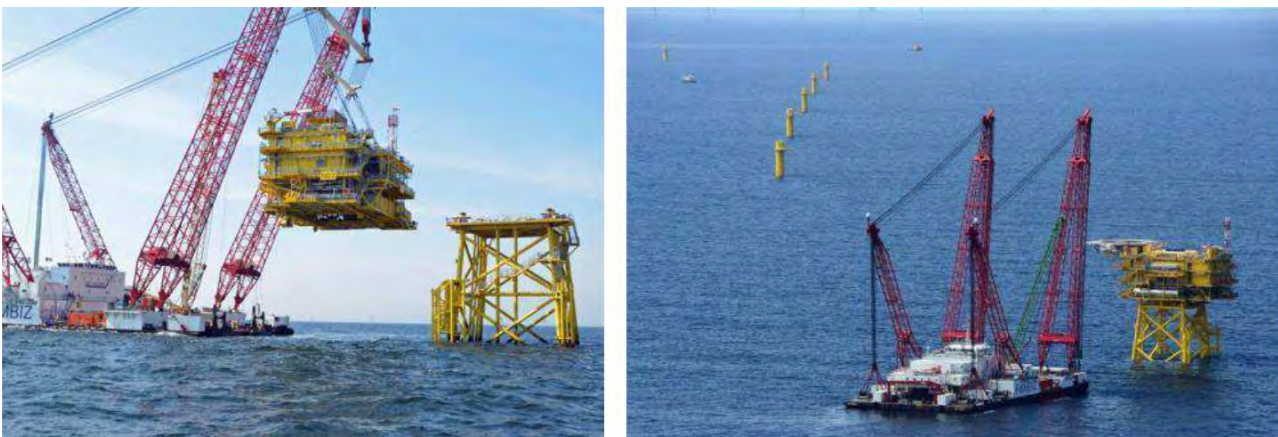
Figure 60 Installation of topside
