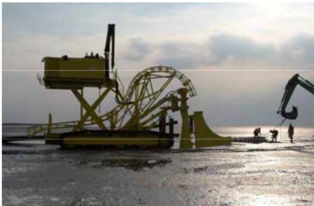
Figure 51 Vibration plough on tracks
