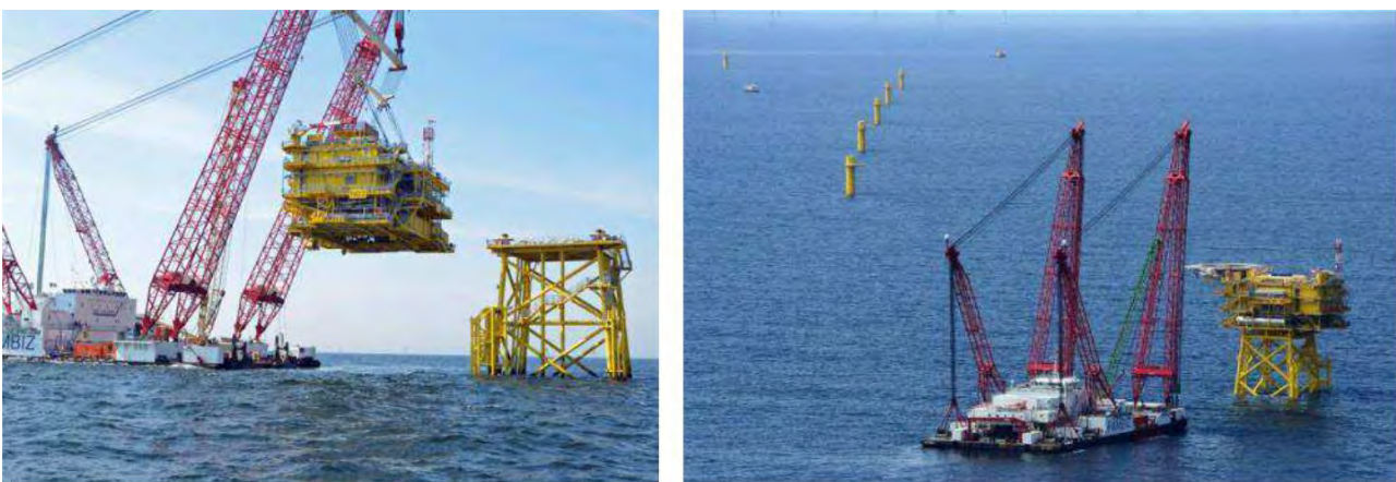
Figure 60 Installation of topside
