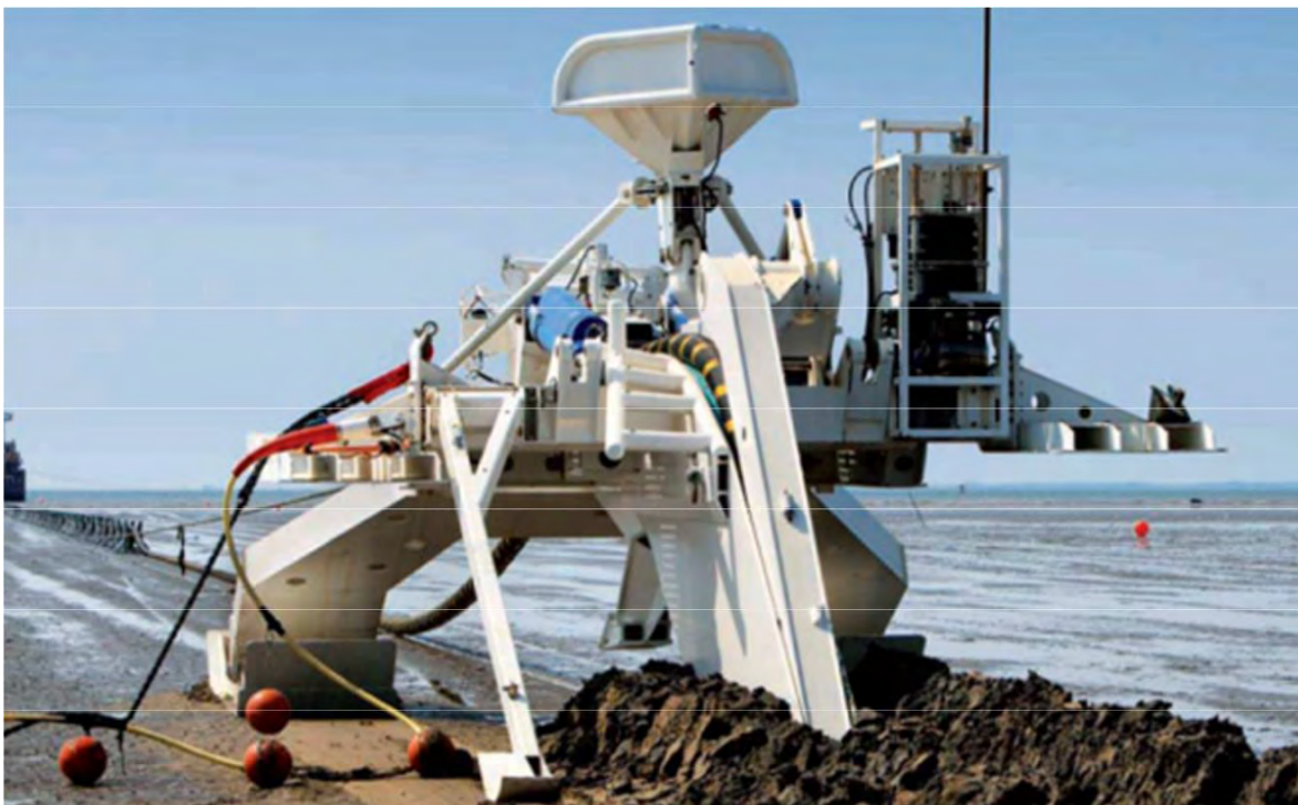
Figure 42 Sea Stallion cable plough
