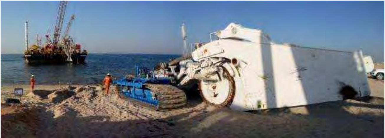
Figure 41 TM04 Wheel cutter cable trencher
