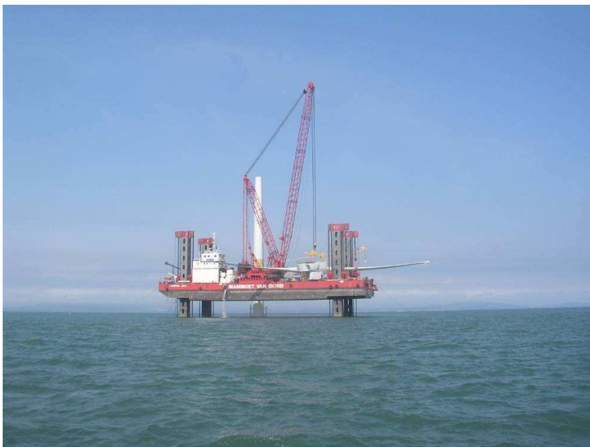
Figuur 4.14 Installatieschip Jumping Jack
