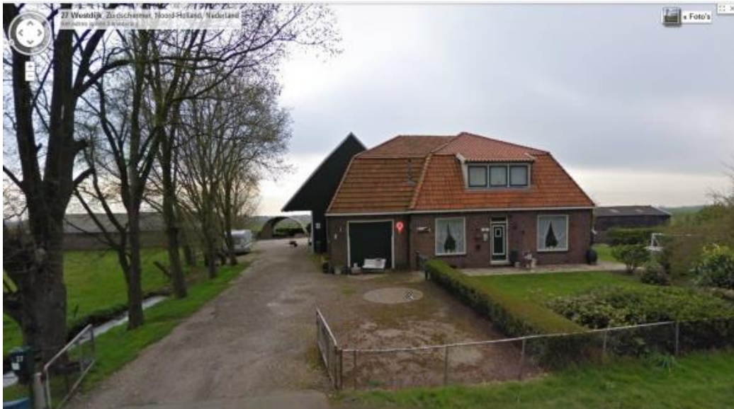
Afb 5: Gebroken schilddak Westdijk 27 (bron: google maps)
