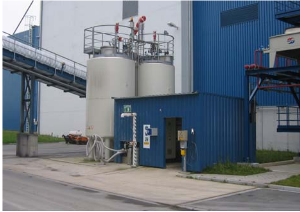
Pic1: Storage tank for ammonia water with pump station
