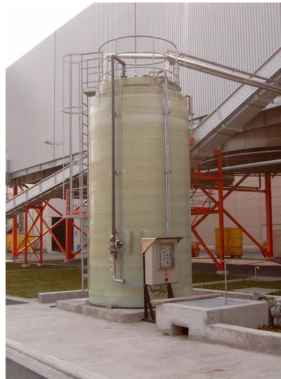
Pic 5: Storage tank and urea solution
