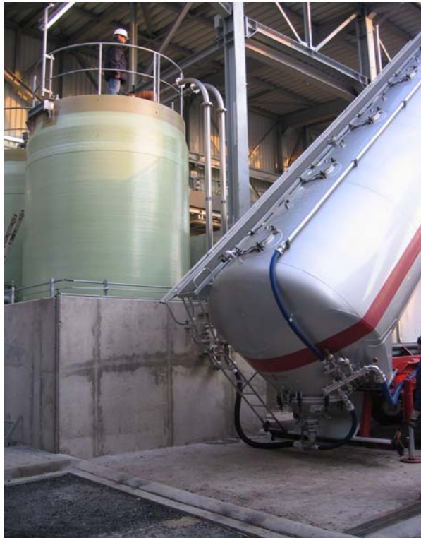
Pic 4: Mix station and storage tank for urea solution
