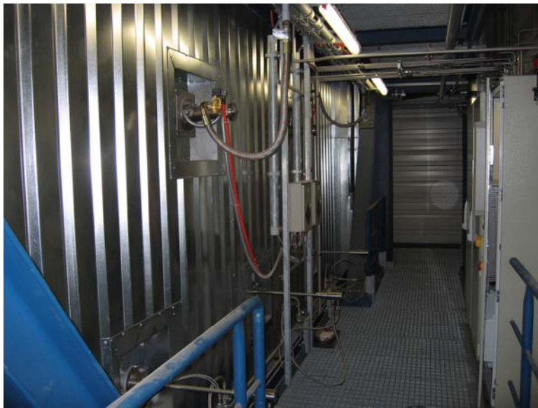
Pic 6: SNCR- Injection's lance with acoustic temperature measurement
