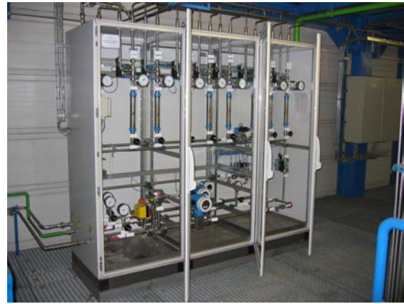
Pic 2: Mixing and metering modul
