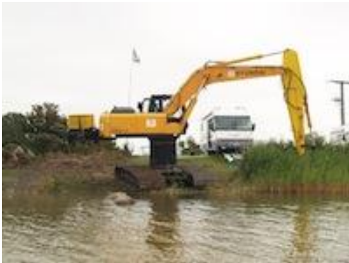
Figure 24: Typical Elevated Excavator
