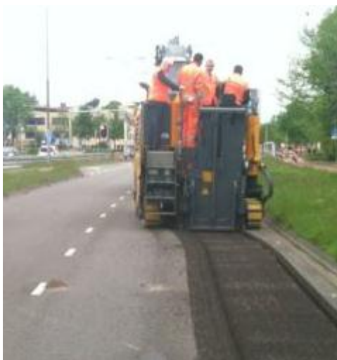
Figure 26: Typical mill equipment
