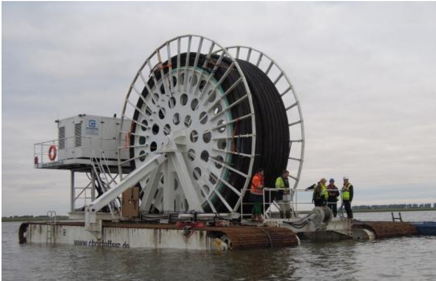
Figure 27: Modular transport vehicle with cable drum
