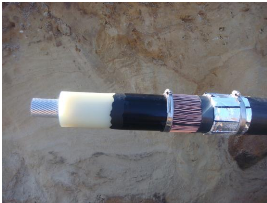
Figure 3: Typical HVAC cable
