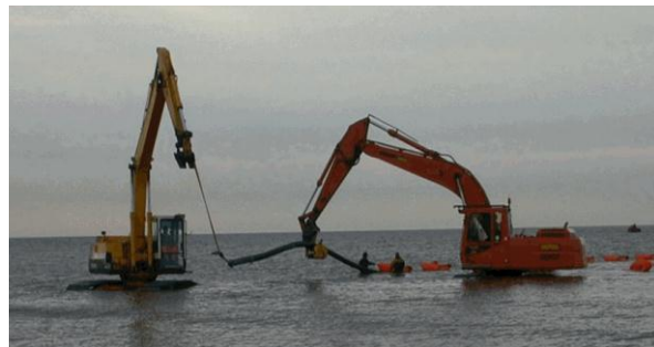
Figure 16: Excavator with lifting bow, removal of floaters
