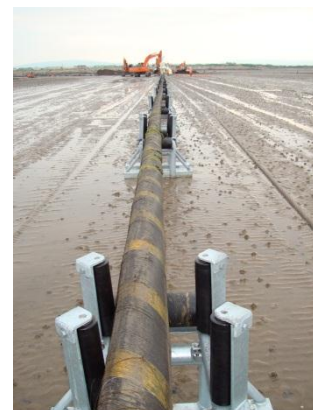
Figure 14: Cable on rollers
