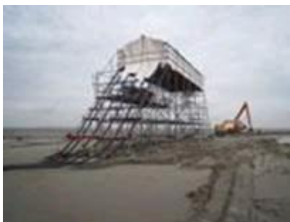
Figure 29: Typical example Shallow water Jointing platform
