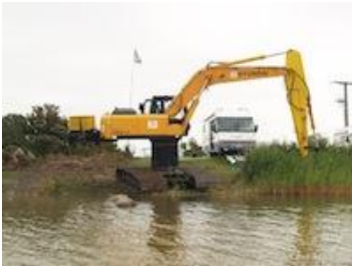
Figure 24: Typical Elevated Excavator
