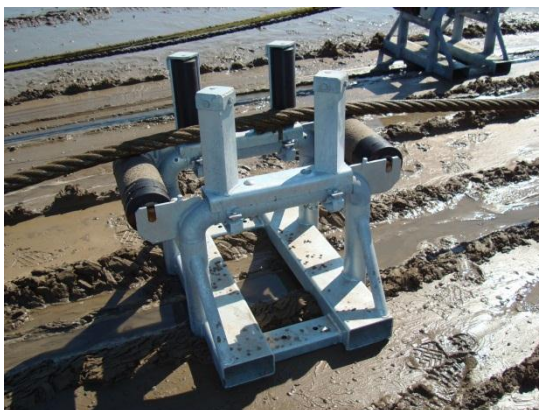
Figure 13: Detail of temporary roller
