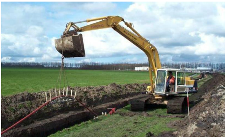
Figure 10: Typical crane with a quadrant
