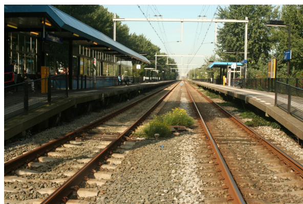
Figuur 4.14 Station Vlaardingen West.
