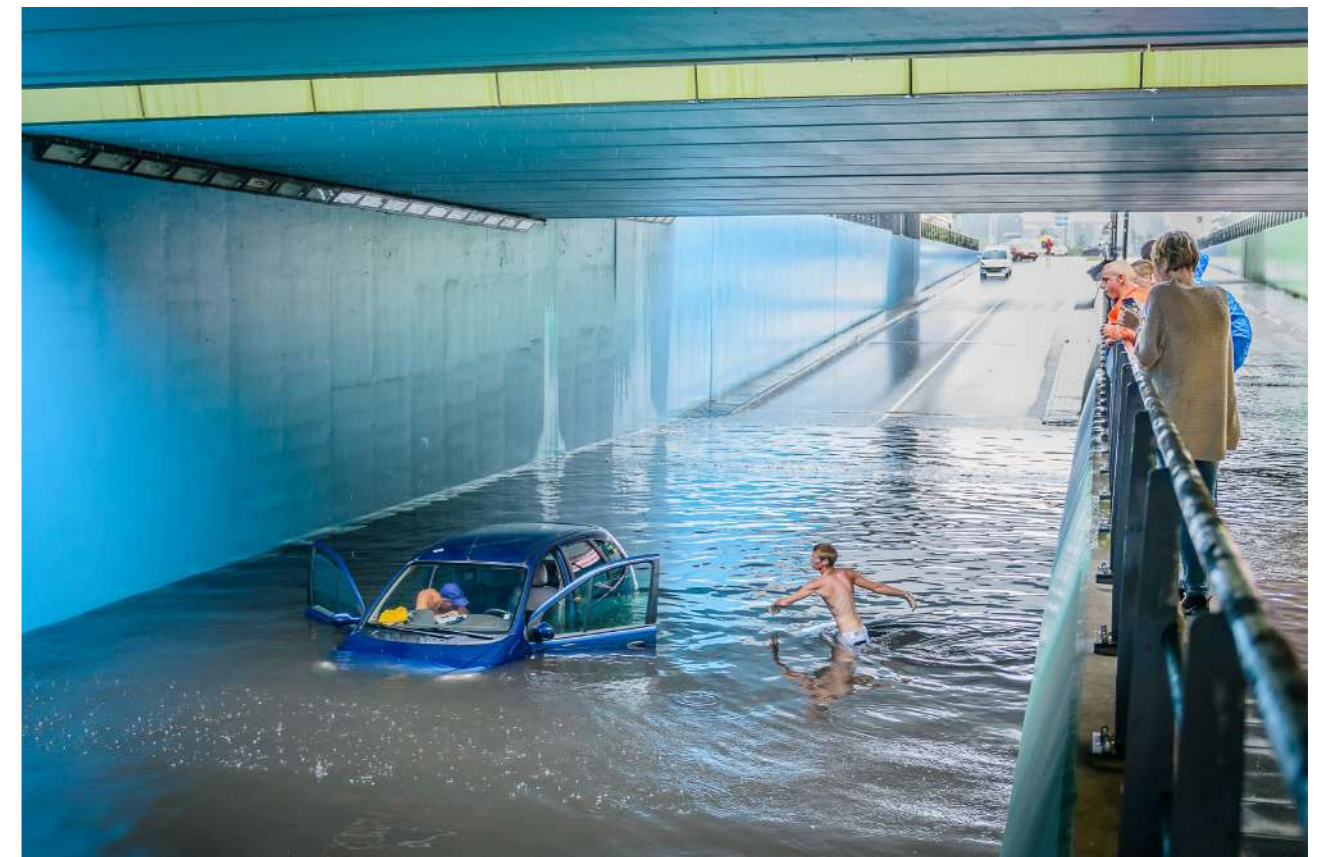
Wateroverlast in tunnel
