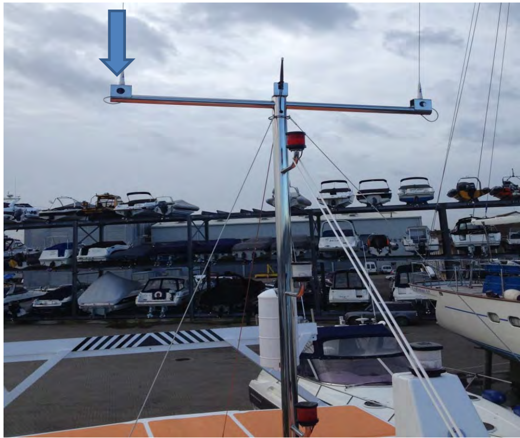
Point 14 – Whip Antenna Base Stbd
