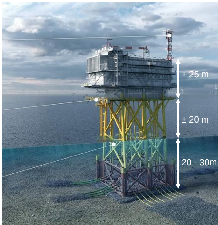
Figure 5 Standardized 700 MW AC offshore substation concept
