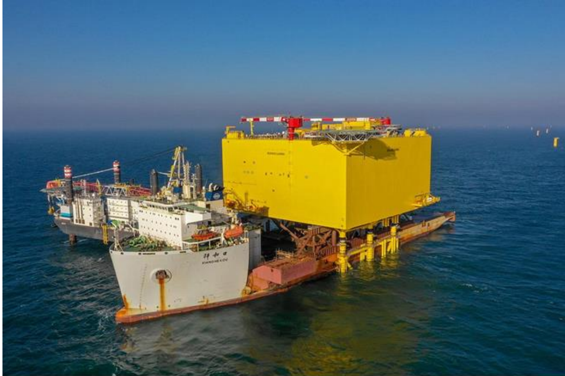
Figure 12 - Float over installation with HTV of the BorWin3 topside
